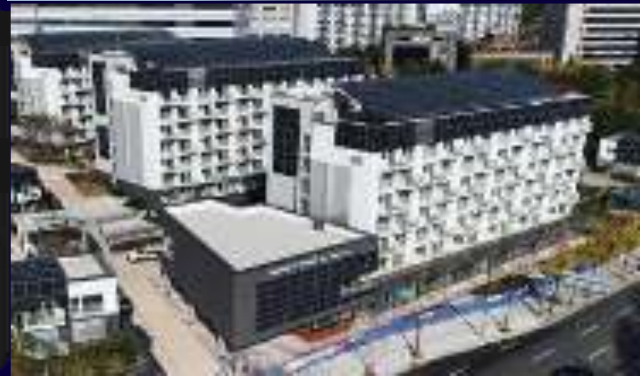
Energy Zero Housing Complex
